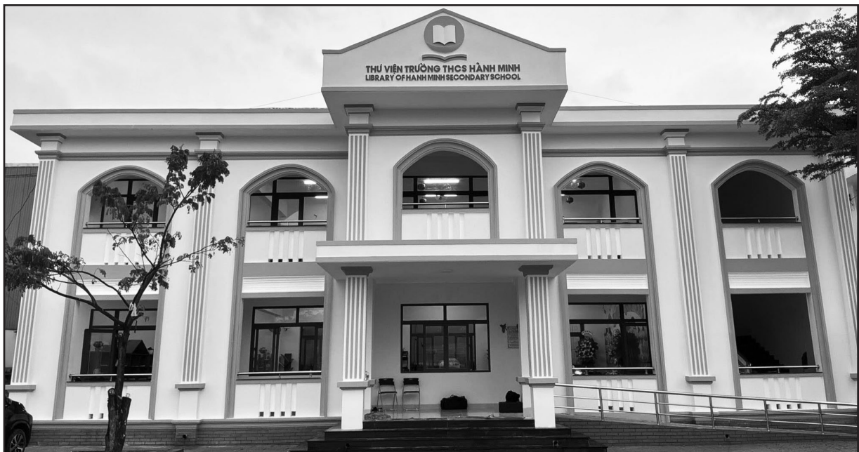
The completed Hanh Minh Library & Learning Center, December 17, 2025.
