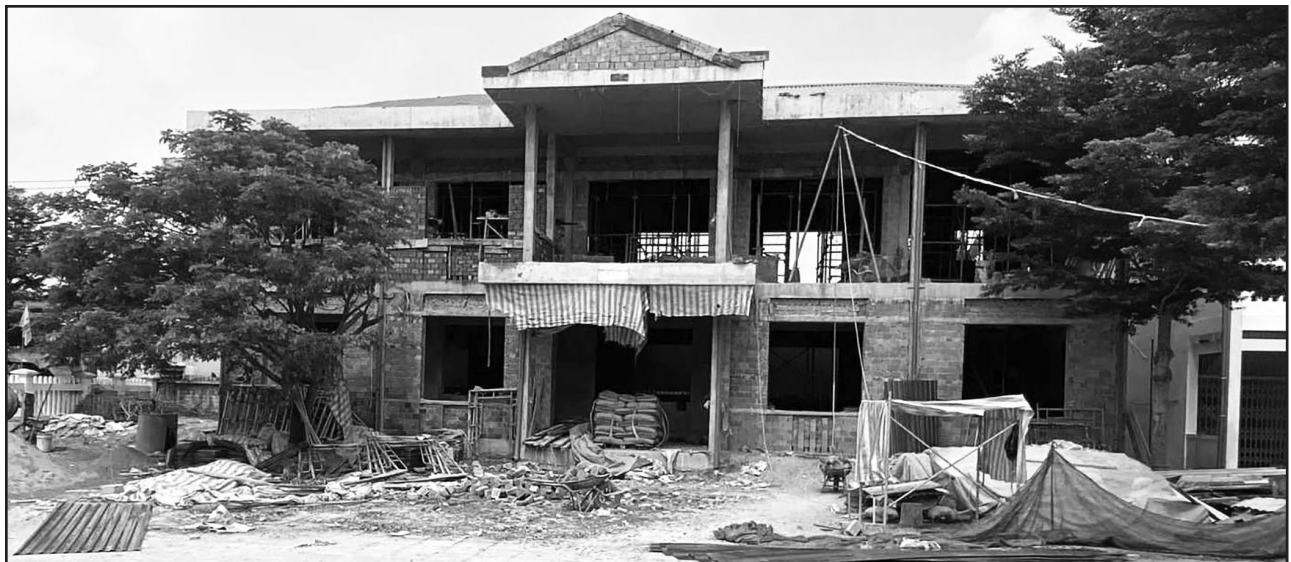
Hanh Minh construction progress as of November 11, 2025.
