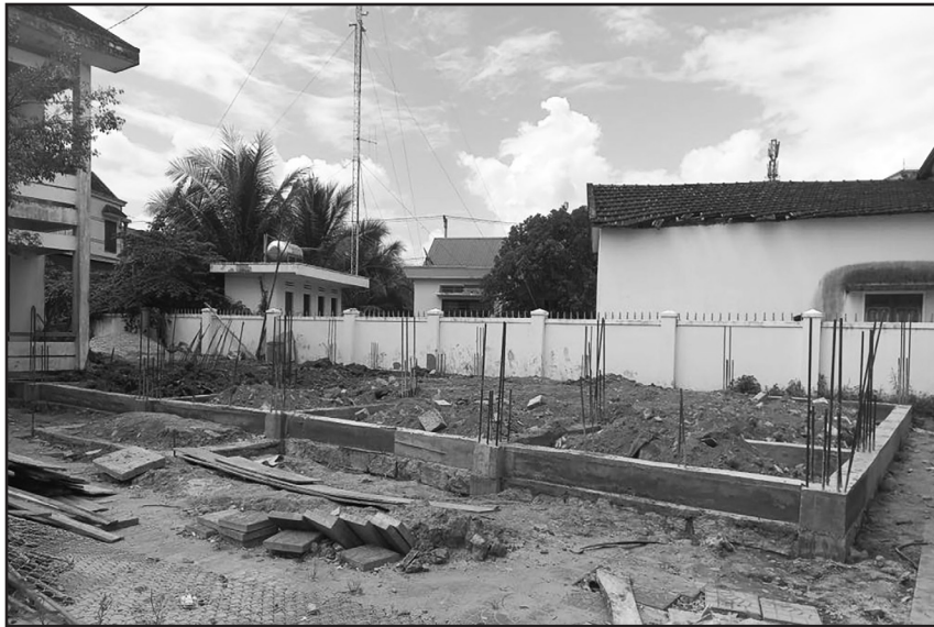
Third VVAW library and learning center under construction.
